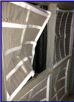
working in just one school. The team also found insulation that had fallen over the heating-cooling vents in the ceiling which stopped air from flowing.
