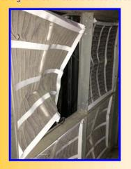
working in just one school. The team also found insulation that had fallen over the heating-cooling vents in the ceiling which stopped air from flowing.
